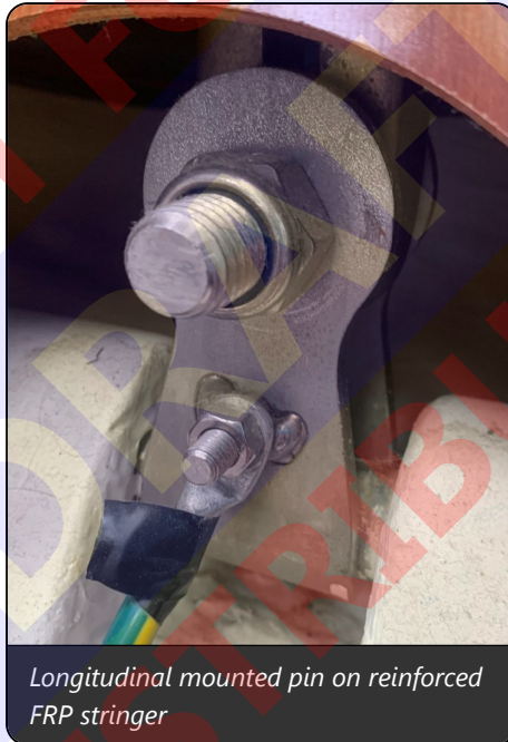
Longitudinal mounted pin on reinforced FRP stringer
