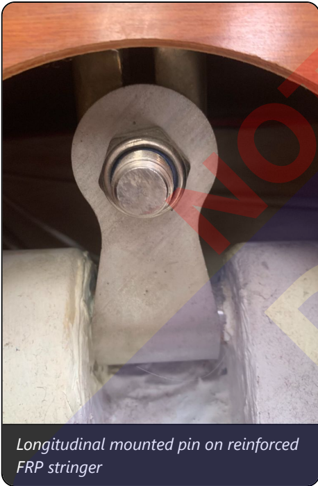
Longitudinal mounted pin on reinforced FRP stringer
